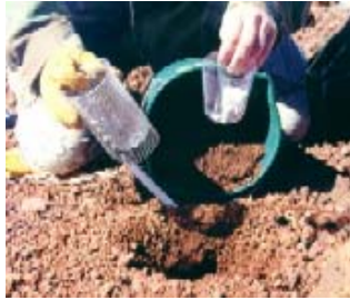
Step 2 Install Wire Tube
