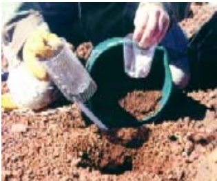
Step 2 Install Wire Tube
