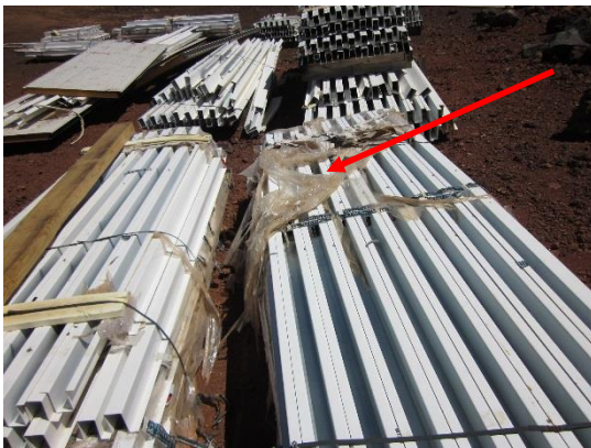
Protective covering on some of the construction material was loose and capable of becoming wind-blown debris.
